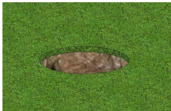
A hole is prepared in the required place in the ground (the hole should be about 80mm larger than the diameter of the box itself, eg for type STAKOHOME-7702-A it is a hole approx. 250mm, as this type has a box diameter of Ø 170mm) and the appropriate cables are fed.
