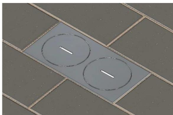
Before the concrete hardens, the floor box is leveled with the ground using a spirit level. Subsequently, the missing tiles will be added.
